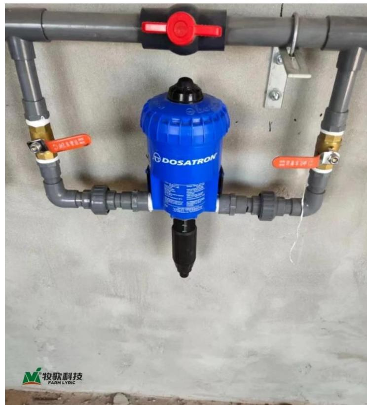
The dosing device can deliver the water soluble medicine into the drinking system to prevent the disease of the chicken. The power is water so no waste of electricity and economical. It is of easy operation and precise control the amount and ratio of the medicine.
